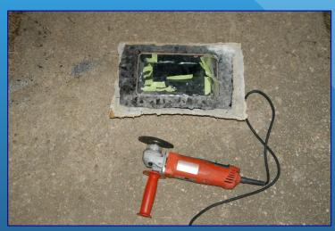
Trim the edges of the mold with a AlO<sub>2</sub> blade on 4-1/2" grinder
